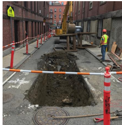
Water and Sewer Installation Sun Court Street
