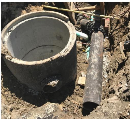
New Catch Basin and Water Main Snow Hill Street
