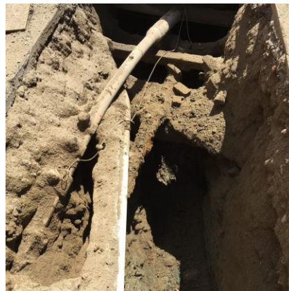
Nearing Completion of Water Main Installation Hanover Avenue
