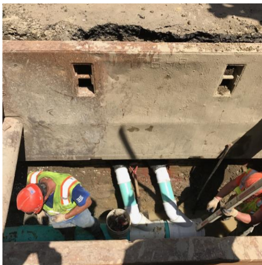
Reconnecting Sewer Laterals Hanover Avenue
