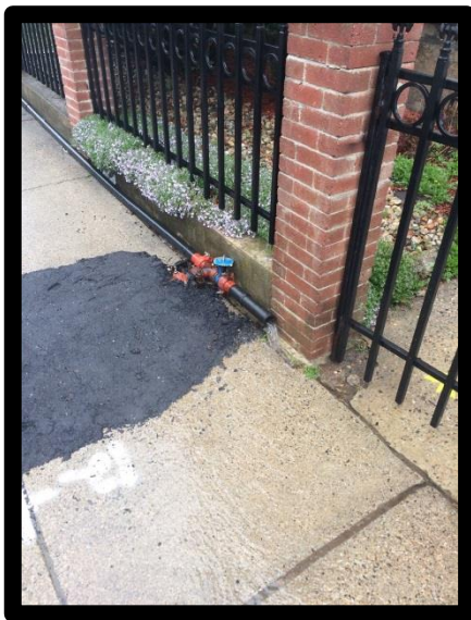
Mount Pleasant Avenue Temporary Water Main Bypass – Chlorinated and Activated
