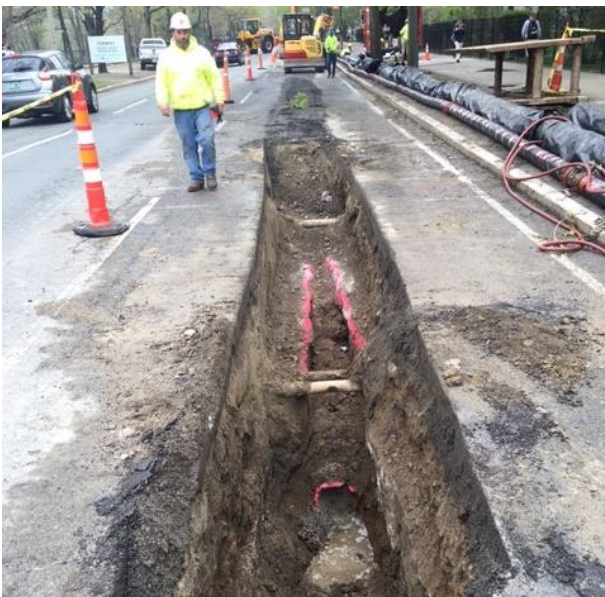
Replacement of Water Main
