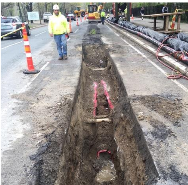
Replacement of Water Main
