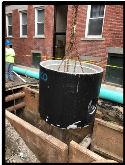
Tileston Street Manhole installation at Wiggin Street
