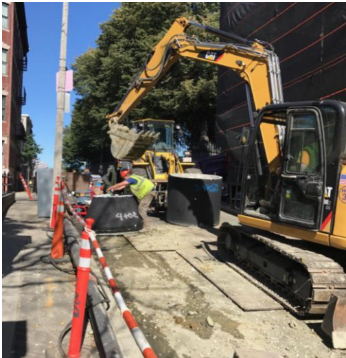
Preparing to Set Sewer Manhole Snow Hill Street
