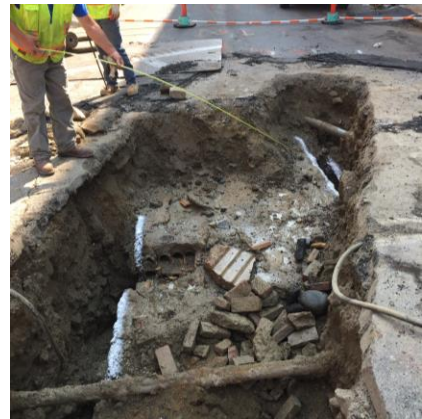
Utility Conflicts Richmond Street at North Street
