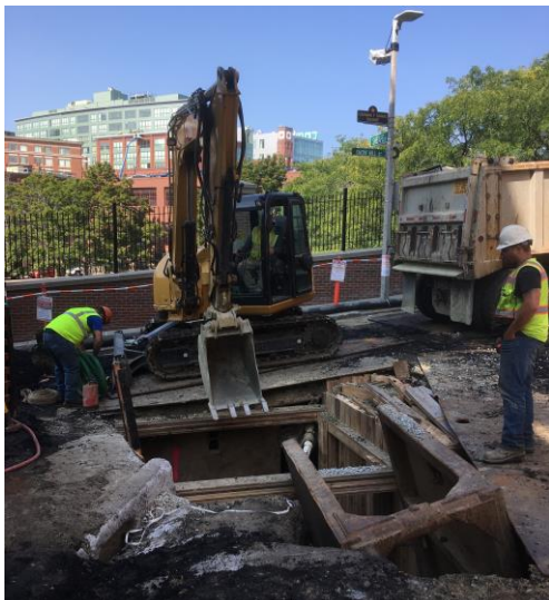
Completing Side Connection with Sheafe Street at Snow Hill Street
