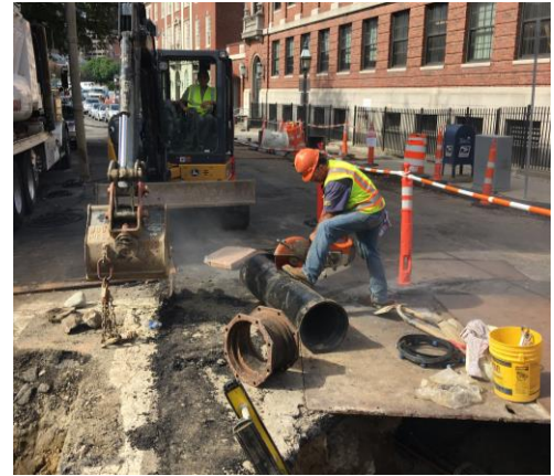
Cutting Water Pipe to Length North Street
