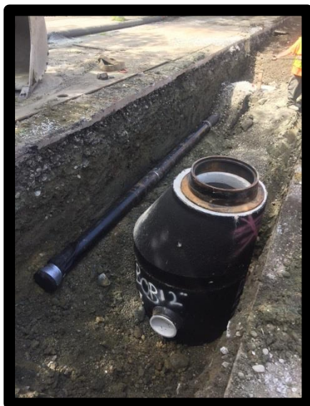
Mount Pleasant Avenue Installing 12" Drain With Manhole and 8" Water Main Pipe
