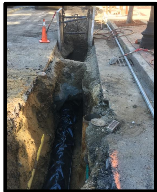
Water Main Installation Warren Avenue at Berkeley Street
