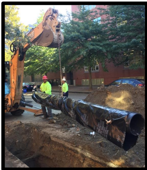
Water Main Installation Warren Avenue
