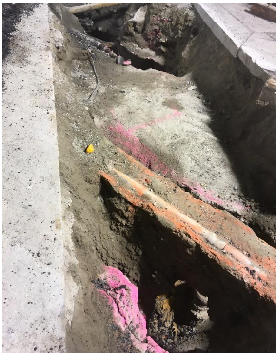
Sewer Replacement Excavation
