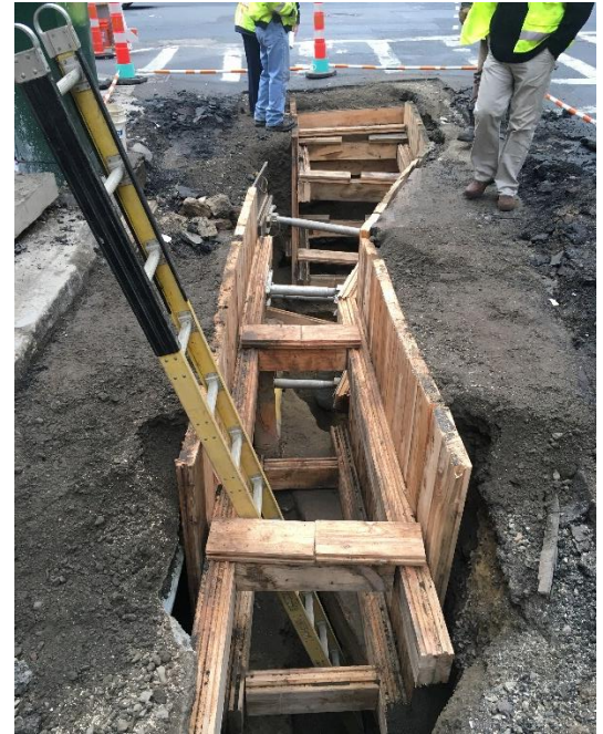
Phase II Excavation
