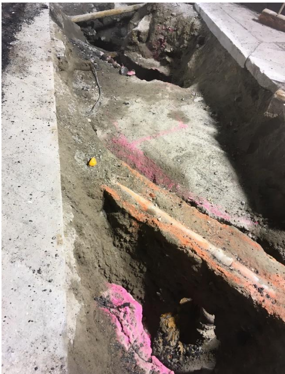
Sewer Replacement Excavation (multiple utilities above sewer)
