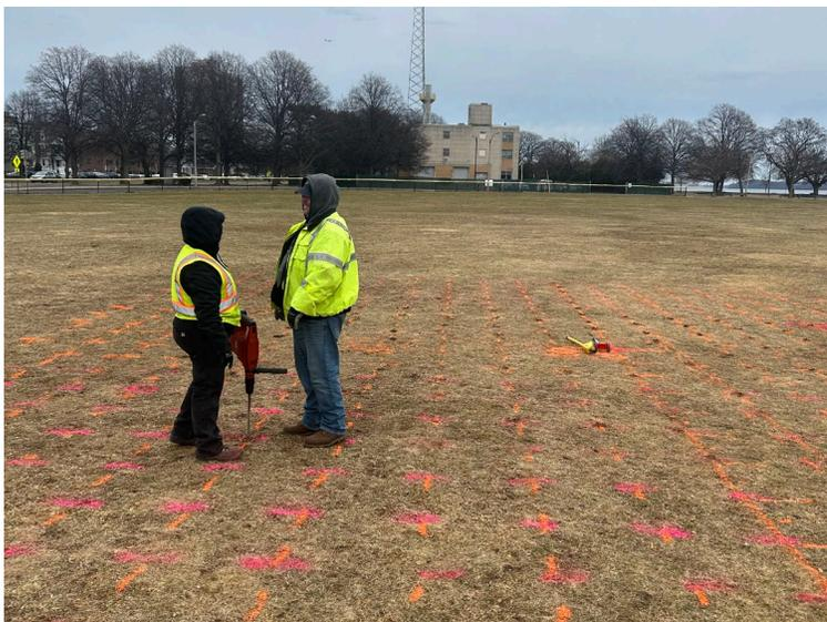
*After crews could not locate buried manhole in Moakley Park by metal detector, a grid was painted to guide drilling exploration.*
