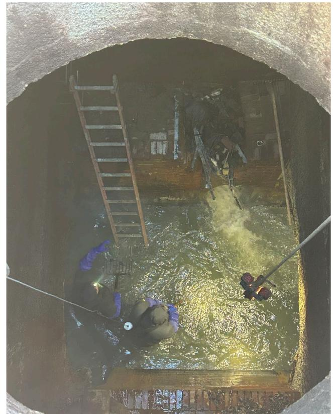
*Initial cleaning of the existing NBMI pipe through Special Manhole B in Moakley Park.*
