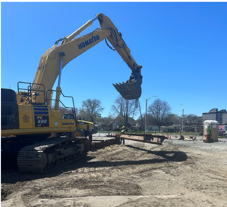
Piles are installed to provide support of excavation.
