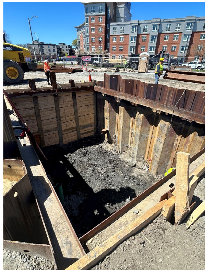
Once support of excavation is installed, excavation begins.
