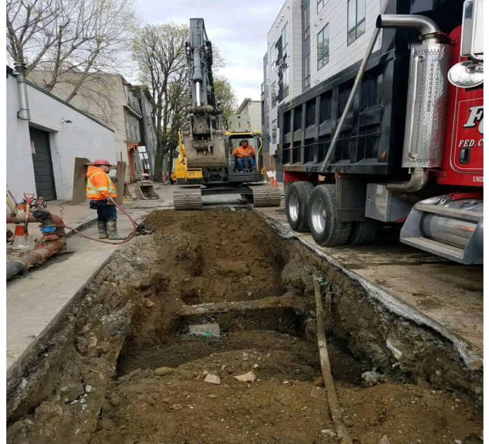
Sewer and Drain Trench Middle Street.
