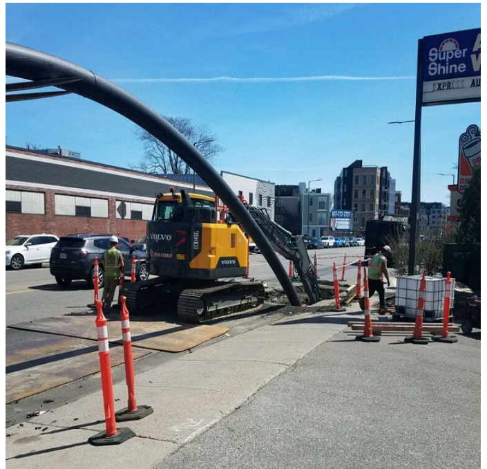
Inserting HDPE pipe bursting Old Colony Avenue.
