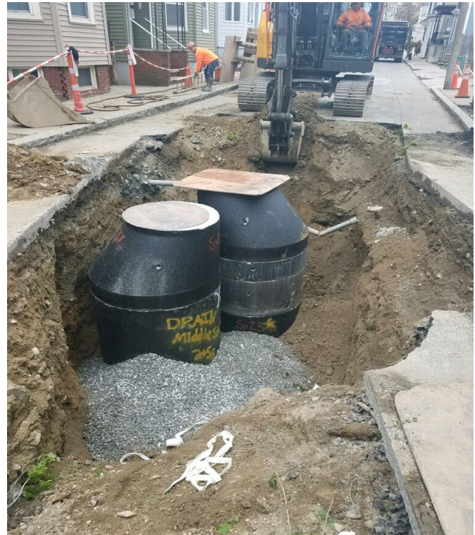
Drain and Sewer Separation Manholes Middle Street.
