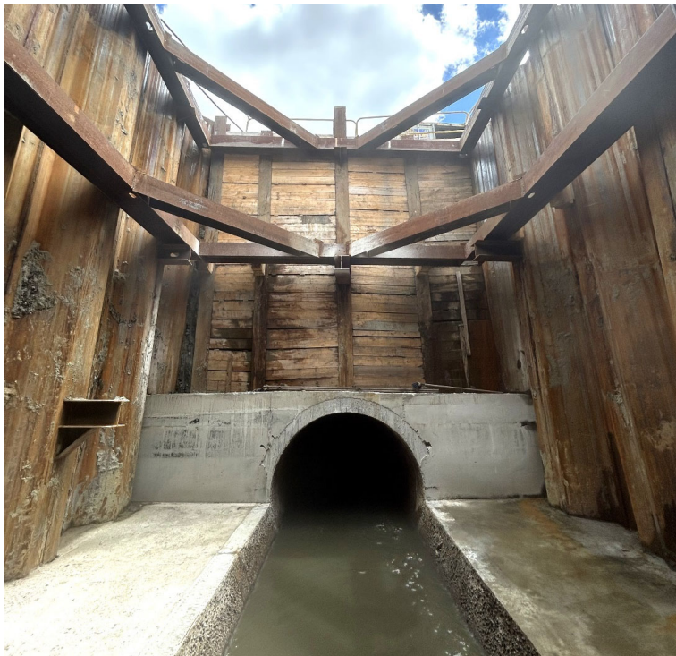
Concrete thrust block collar installed around the pipe.
