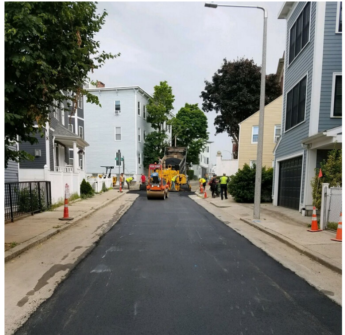
Temporary paving on Middle Street
