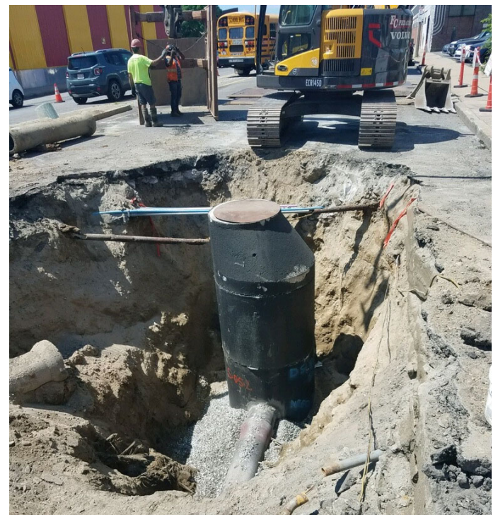
Sewer Manhole on Old Colony Avenue at D Street
