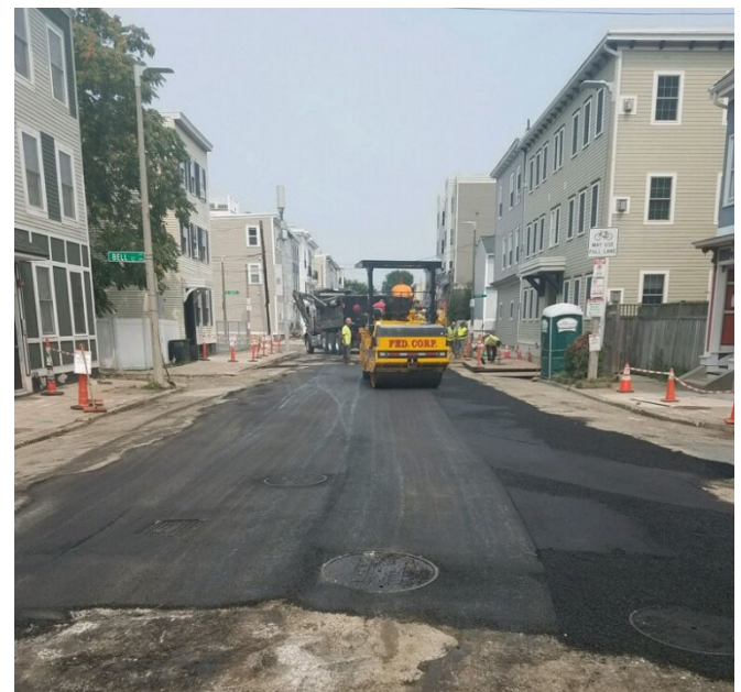
Temporary paving of D Street at West Ninth Street
