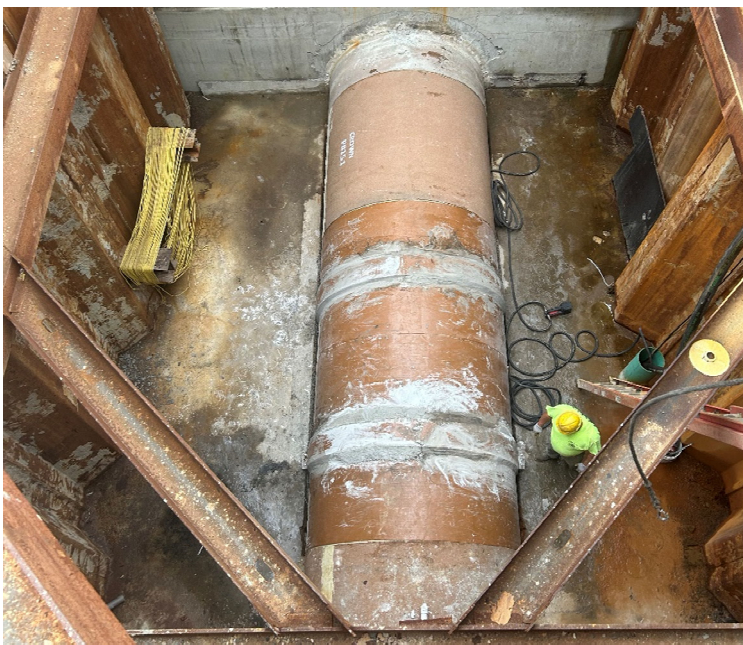
Closure of slipline pipe in access shaft.
