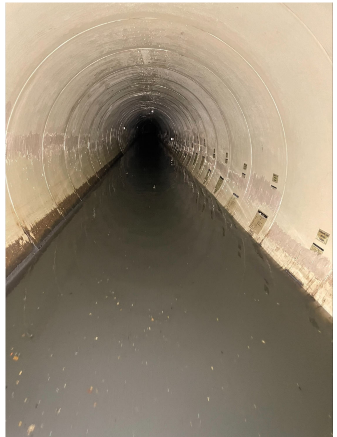
Completed sliplining of NBMI.
