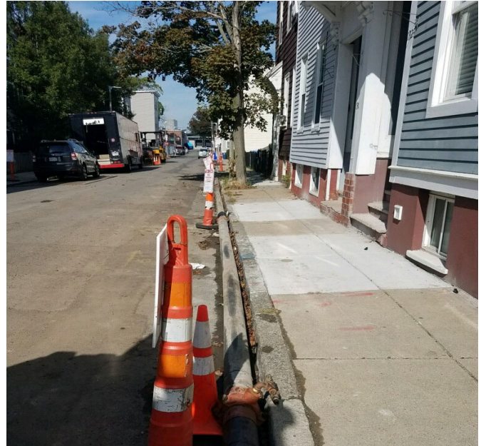
Temporary Water Bypass West Eighth Street
