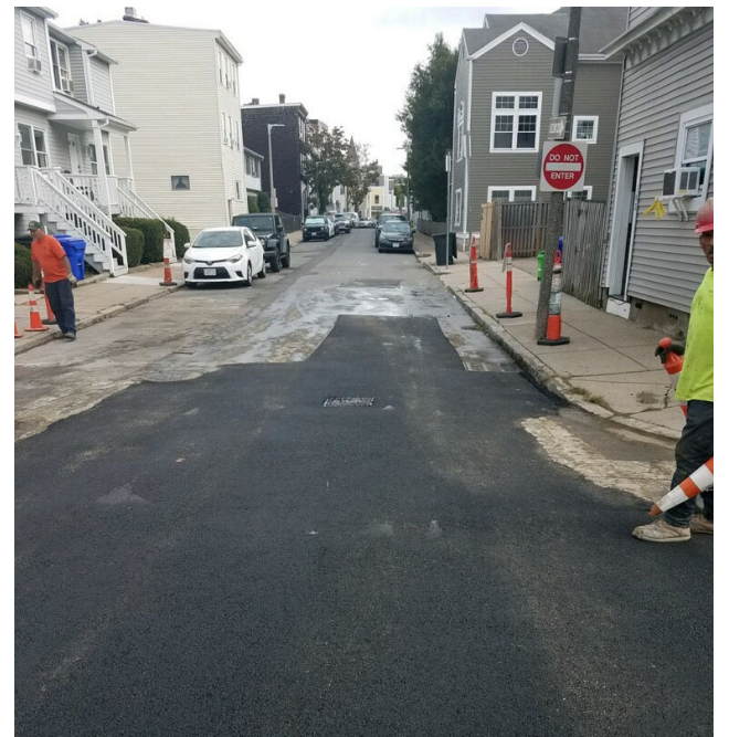
Temporary paving of D Street at West Eighth Street
